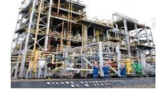
Polypropylene plant at Refinery Unit III, Plaju
